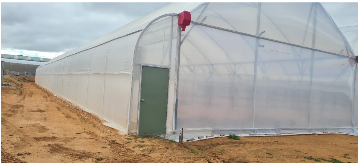
Insect screen over exhaust fans – doors are emergency exits only
