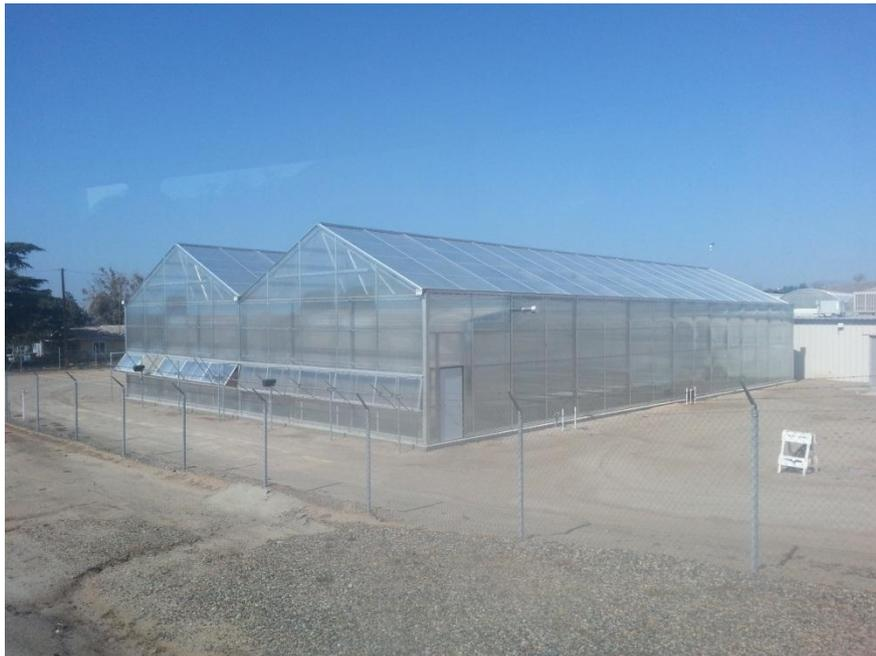
**Figure 1 - A positive pressure insect proof greenhouse at University of California, Riverside Ca.**
